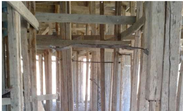
Formwork Of Traditional System Slab
