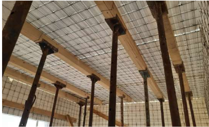
Formwork Of Zenon Panel Slab
